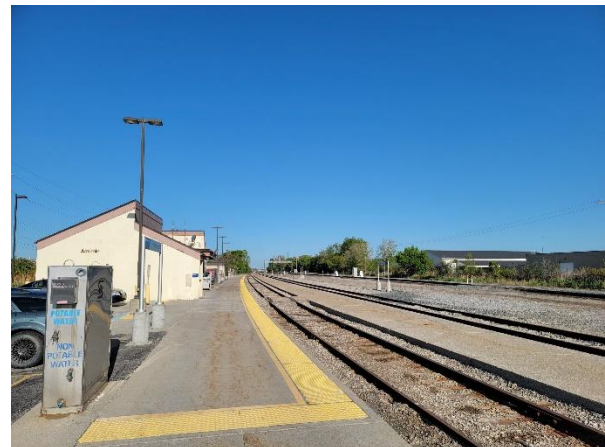
Figure 3: Existing Station (North Side)
