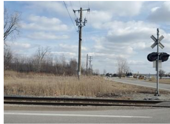
Figure 19: Overhead Lines at Dove St. and 32 nd St.
